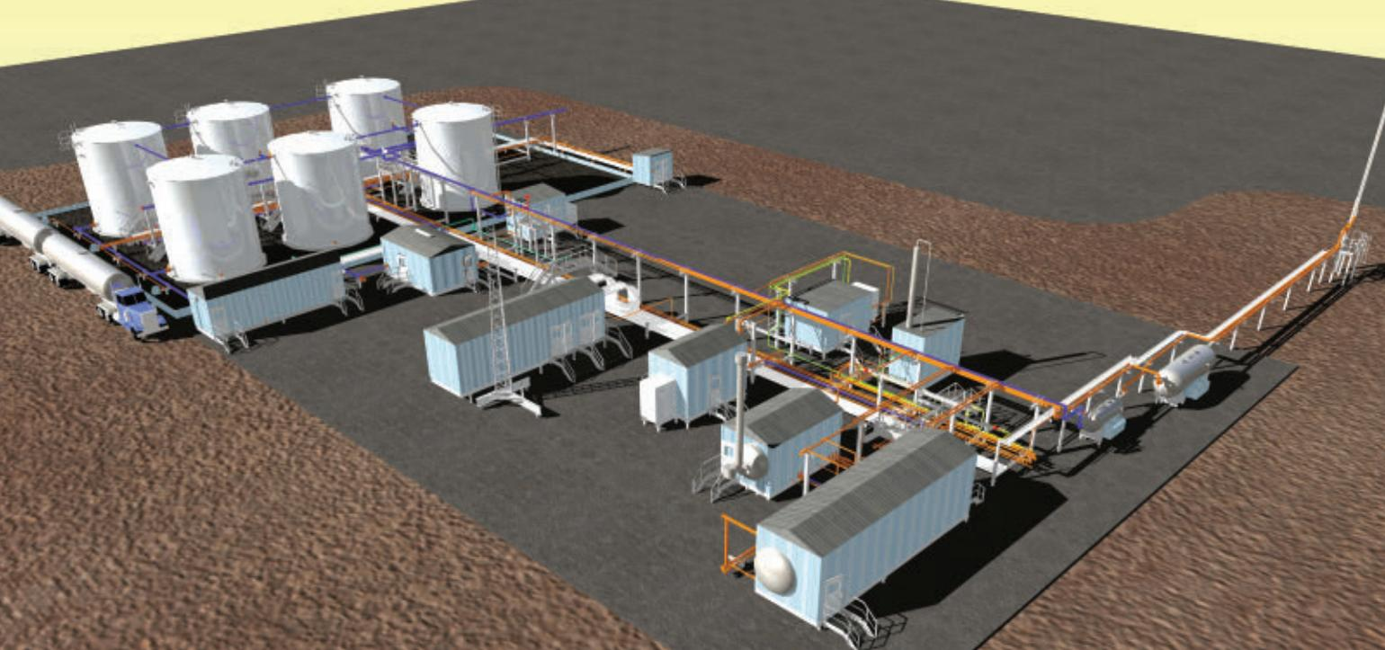
The crude oil and solution gas from the Bakken formation is delivered to free water knockouts and then to an oil battery (as shown in this image).
